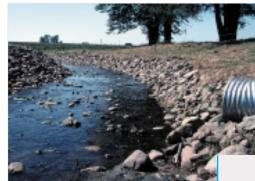
This stream bank has been stabilized and protected from erosion by riprap. Photo courtesy of the NRCS.
