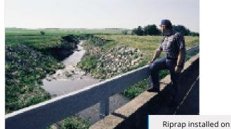
a stream bank helps control livestock access and minimize erosion. Photo by Lynn Betts, NRCS.
