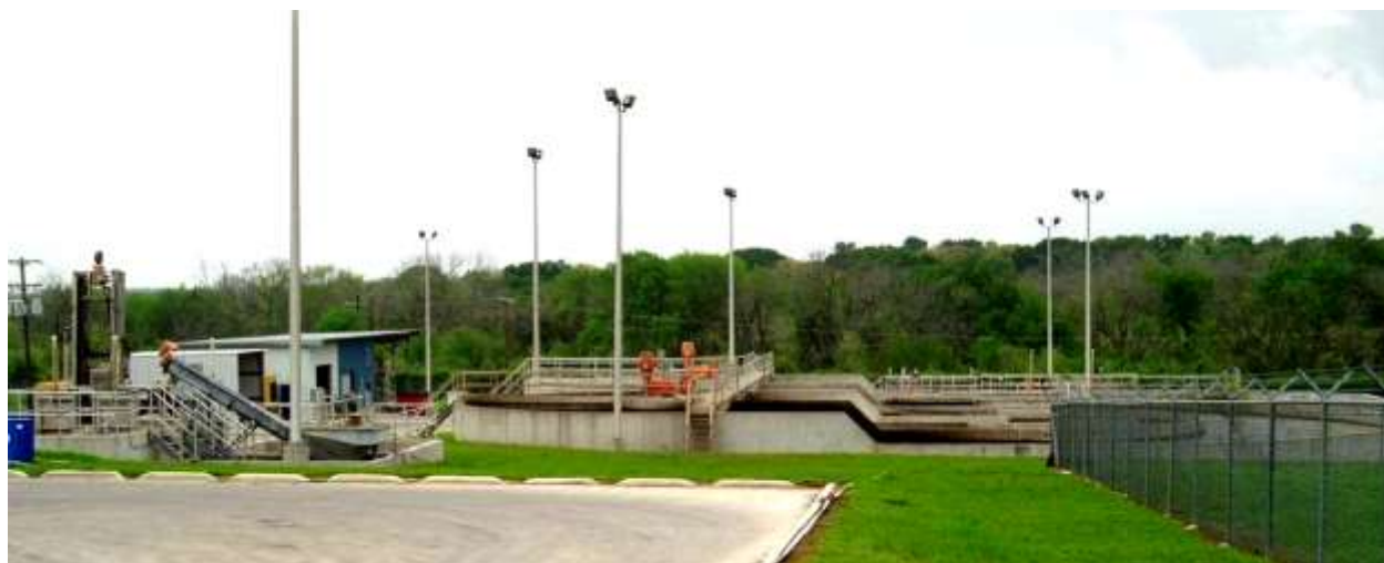
Figure 6.8. City of Lockhart Wastewater Facility No. 2 is managed by the Guadalupe-Blanco River Authority and utilizes UV sterilization to treat bacteria in wastewater.
